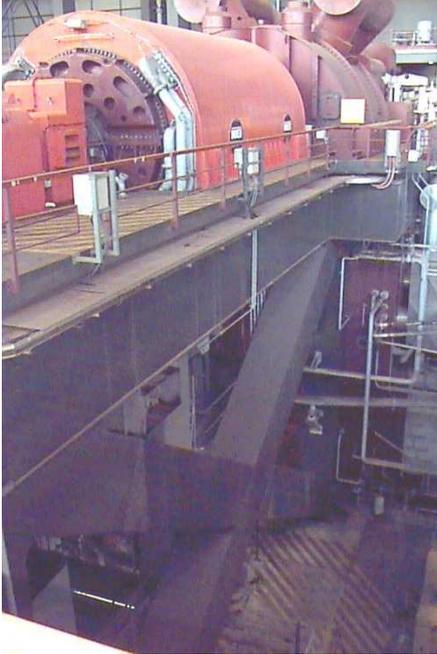
Fig. 2 Flexible steel-beam foundation for earthquake protection
